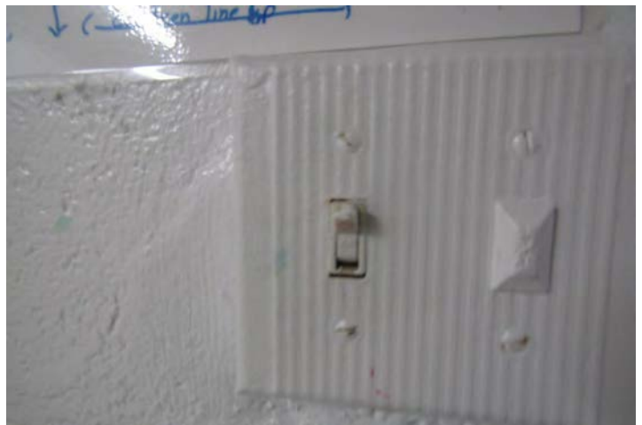
Switch plat and switch has been painted
