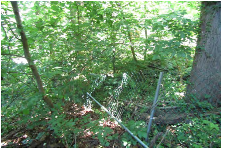
Chain-link fence is damaged
