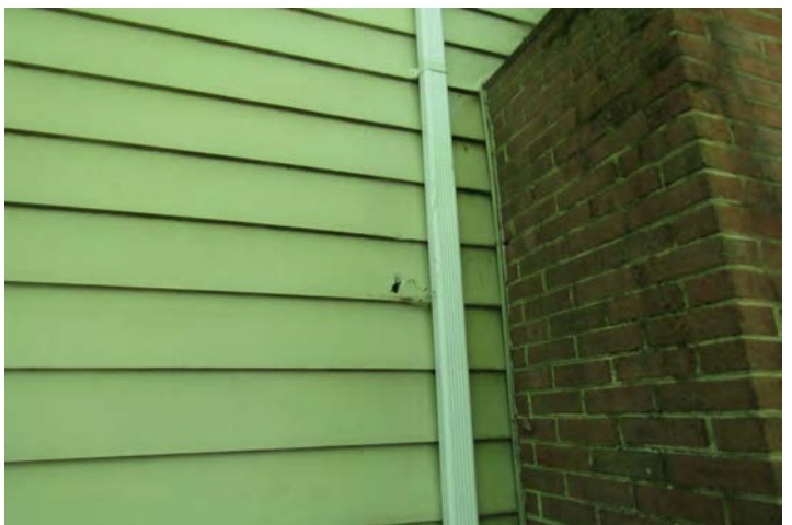
Siding damage
