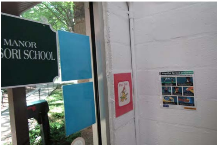
Debris buildup in the corner
