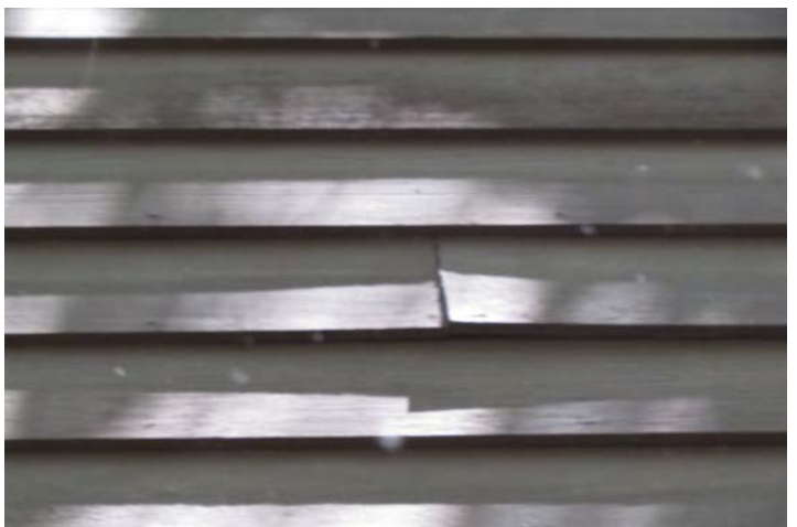
Warped siding
