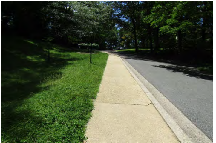
Sidewalk needs safety bollards and handrails
