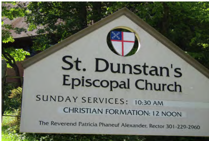
Monument sign needs repainting
